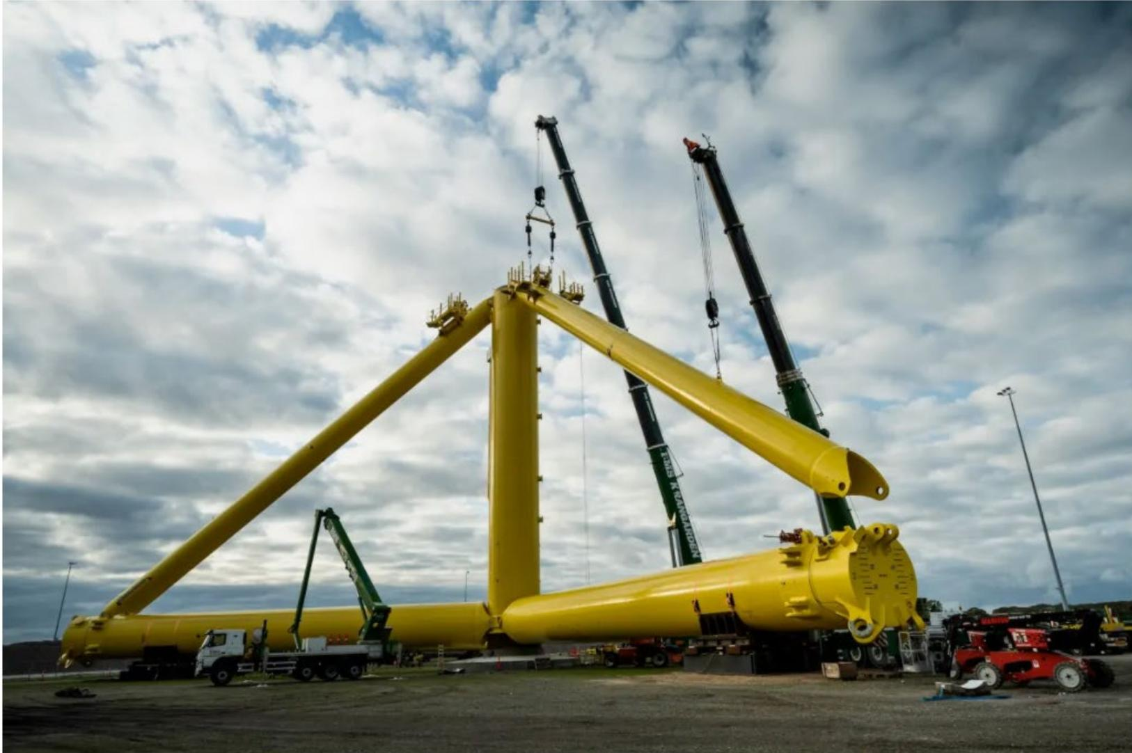
Mounting of the diagonals using maintenance-free proprietary technologies for fast assembly.
